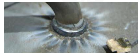
Drawn-arc stud welding in progress - completed 360^\circ weld collar
