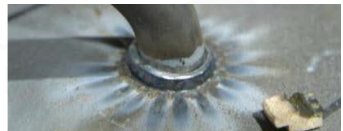
Drawn-arc stud welding in progress completed 360° weld collar
